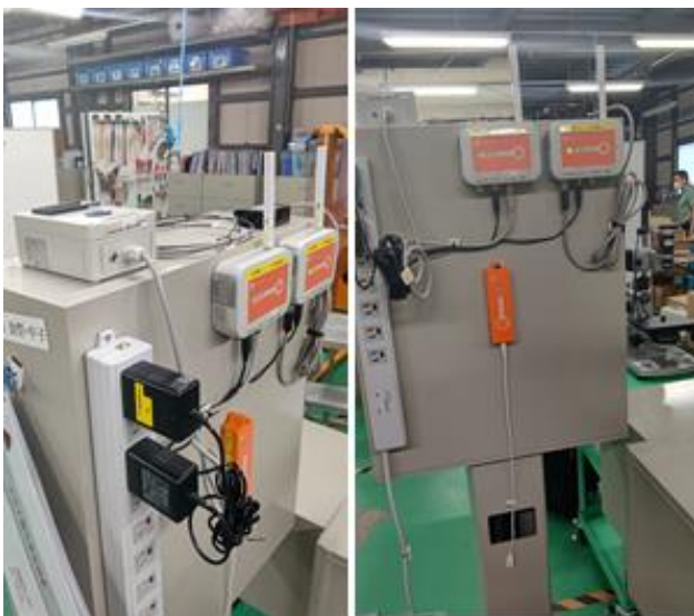
Fig.4 Test operation at head office of Himecs, Inc.
